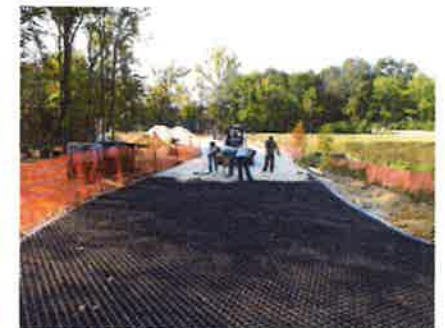
Grasspave2 product being installed in a fire lane.
