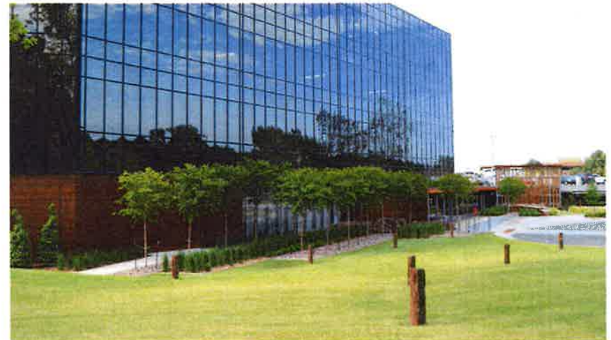
Grasspave2 Fire Lane approved and installed at the Society of Geophysicist Corporate Headquarters, 8801 S. Yale in Tulsa, OK.
